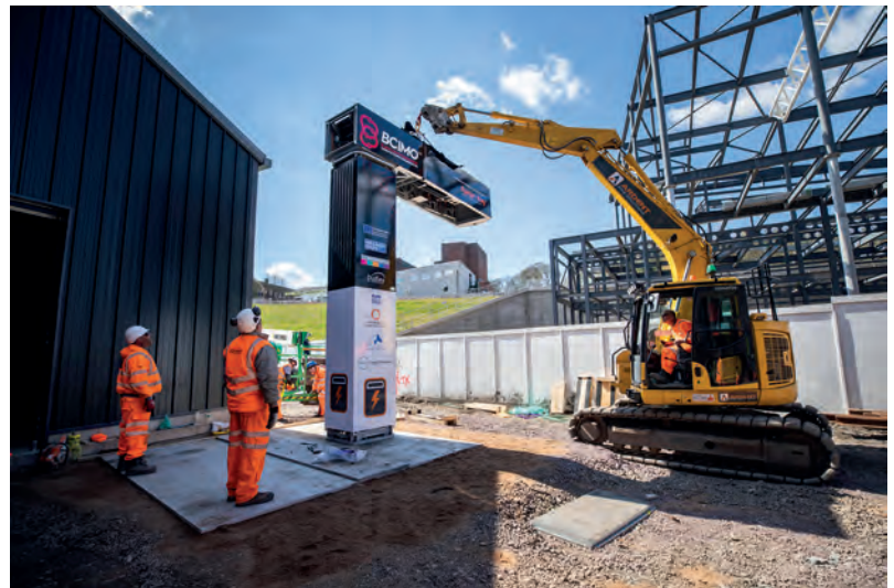
Figure 8: Charger installation with gravity pad (Photo: Furrer+Frej).
