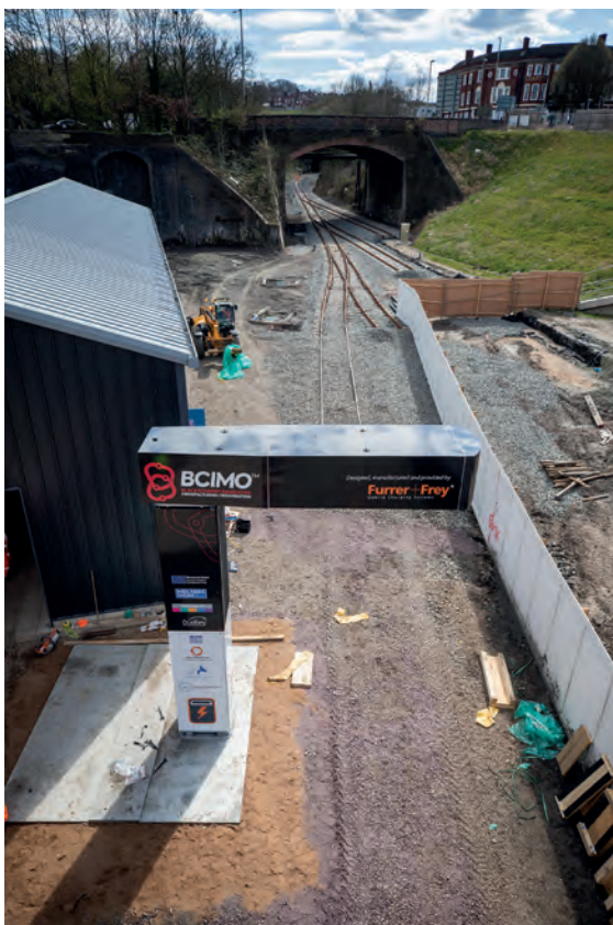
Figure 9: Initial Track location prior to the charger installation (Photo: Furrer+Frej).
