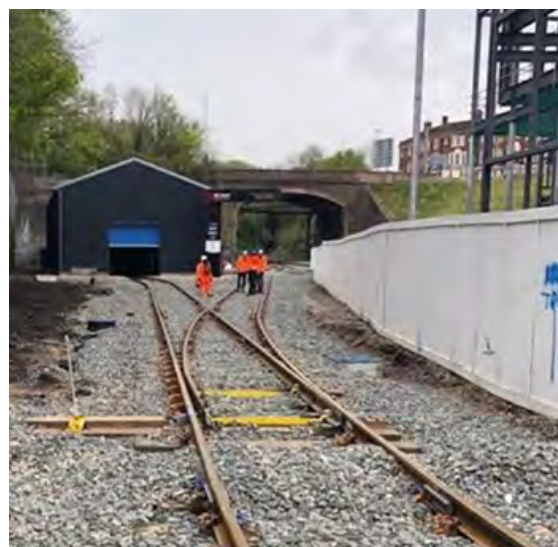
Figure 10: Charger location (Photo: Furrer+Frej).
